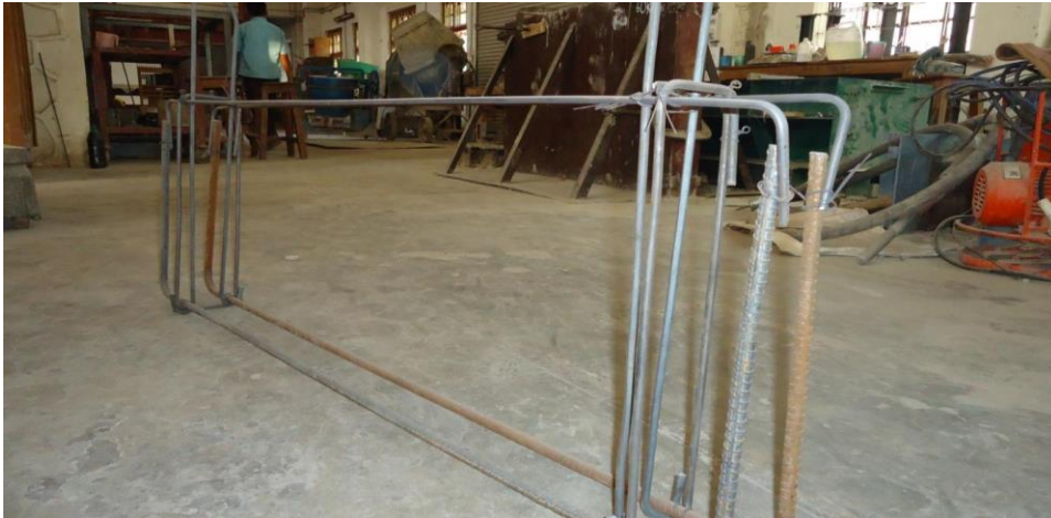
Reinforcement cage
